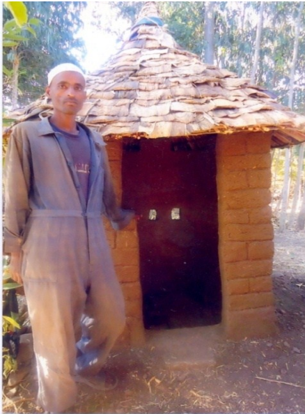
Fig.5: Toilet constructed by the one of the SRDU trainees as seen in the picture
