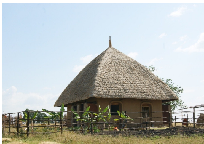
Fig.1: The completed SRDU
